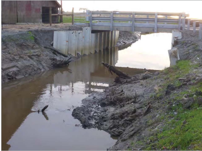
Figure 4. Slumping bank along the right side of the channel immediately upstream of the new bridge and sheet pile retaining wall at Station 14+00 on the profile.
